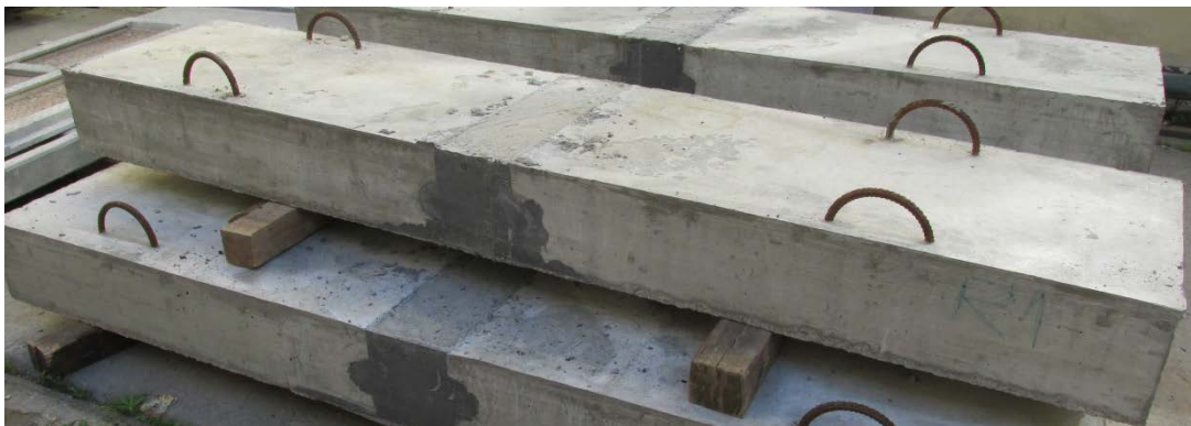
Fig. 1: Precast concrete deck with UHPC joint
